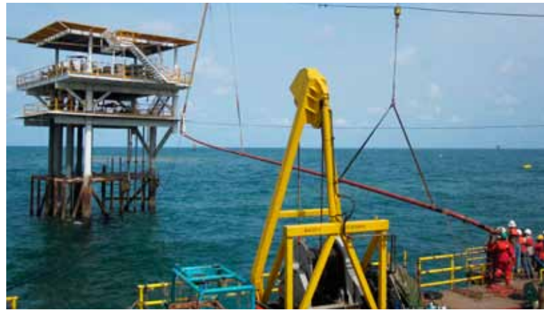
Stalk-on riser installation
